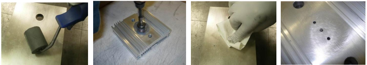
(a) Contact grease is applied to the surface sparingly (b) Abrasion of the heatsink using contact grease and rotating wire brush (c) Cleaning the surface right before mounting the disc (d) Mounting surface, lightly abraded
